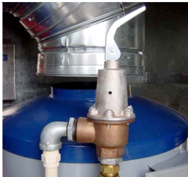
Fig. 6 Temperature & Pressure Relief Valve - Open
