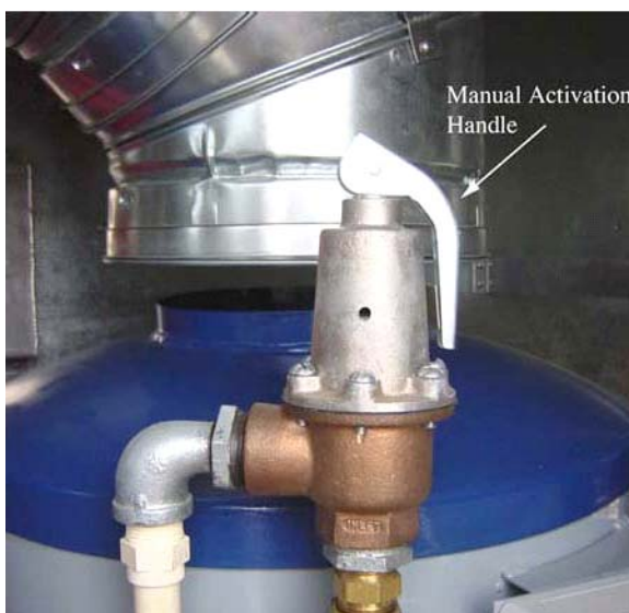
Fig. 4 Temperature and Pressure Relief Valve
